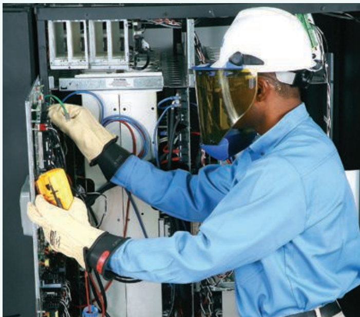
Proper preventive maintenance reduces the risk of UPS failure through thorough inspection, cleaning, testing and calibrating various electronic and mechanical components.
